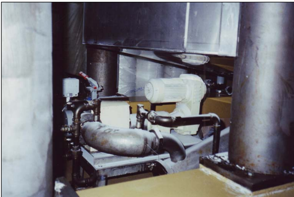
Series S3 pump transferring vegetable fat in UK
